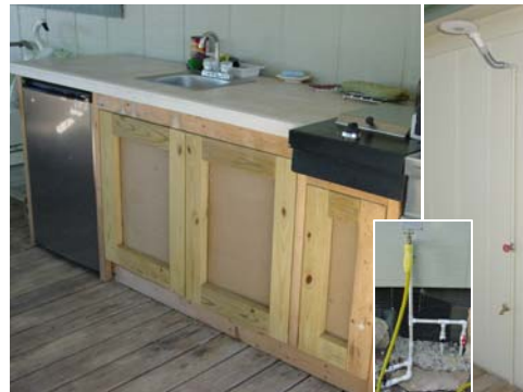
March-May deck kitchen, pool shower, yard water plumbing project
